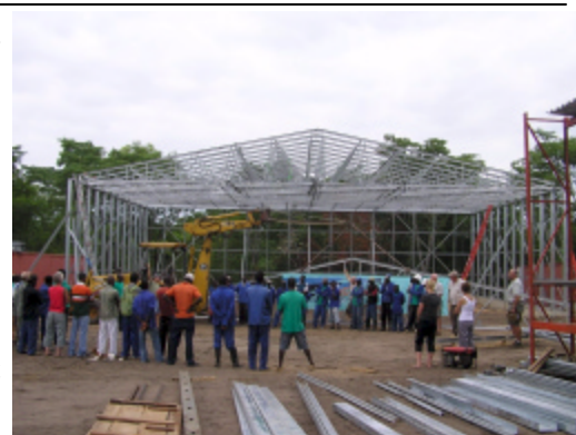
The hangar under construction
